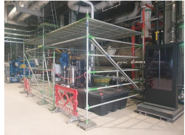
Scaffolding built over and surrounding equipment to protect it from damage.
